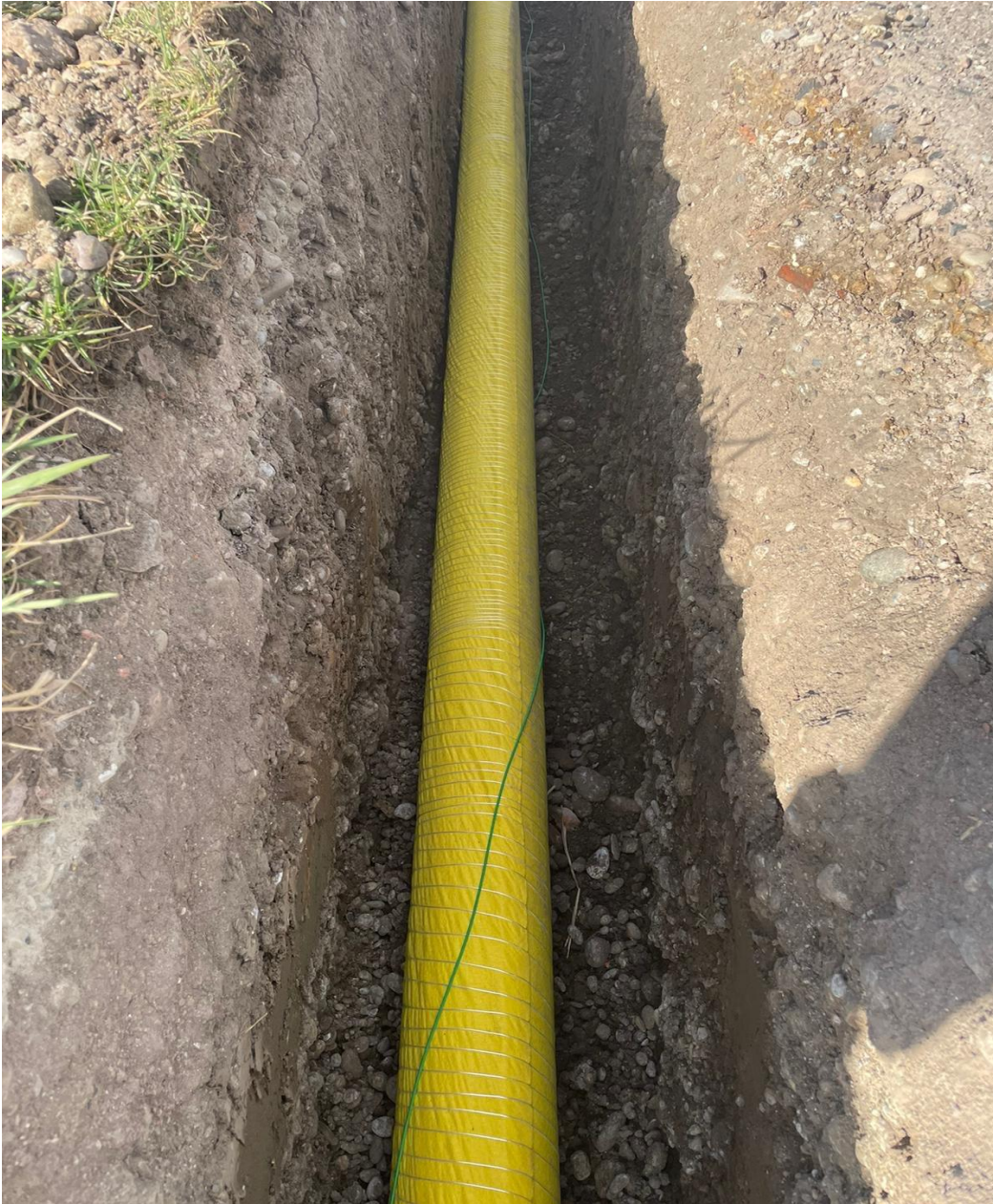
Gas pipe with a tracer wire attached.
